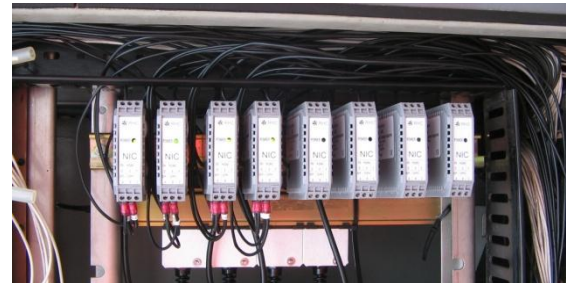
Hall Effect transducers measuring track circuit receiver current.
